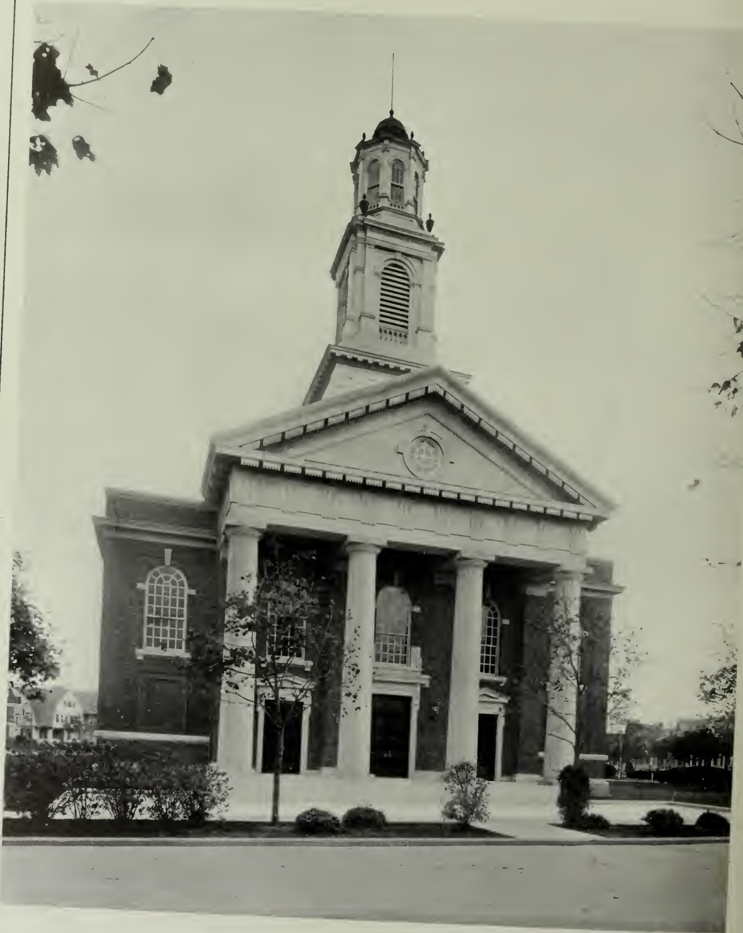
FLATBUSH CONGREGATIONAL CHURCH, FLATBUSH, L. I., N. Y. ALLEN & COLLENS AND LOUIS E. JALLADE, ARCHITECTS.
